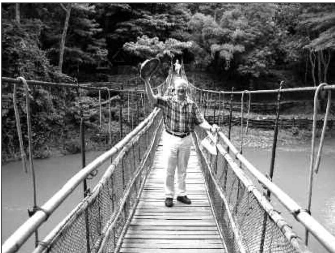
Cal Roetzel on a bridge crossing the Kok River located in the Northwest Region of Thailand.
